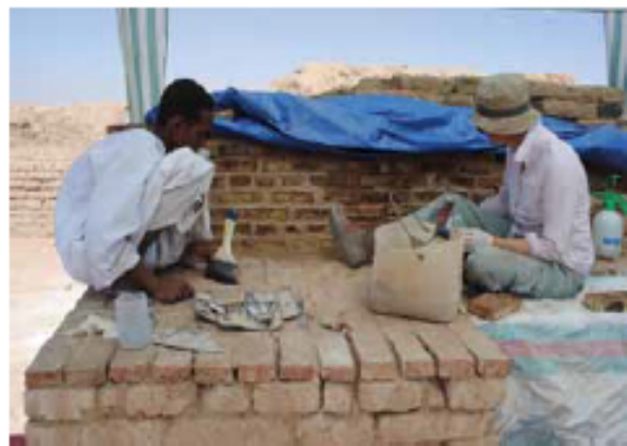
Fig. 10: Building up the vertical wall
