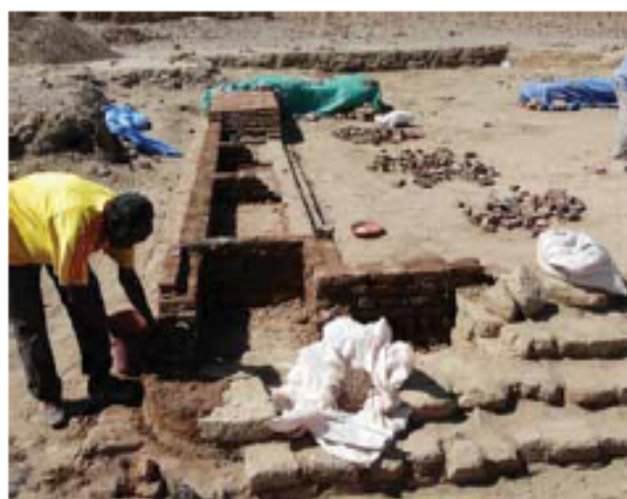
Fig. 16: Brick capping the Kiosk walls, 2011.
