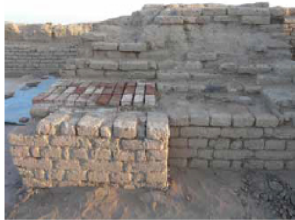
Fig. 8: Capping exposed walls
