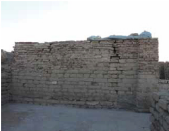
Fig. 11: Failed pointing to capped wall.
