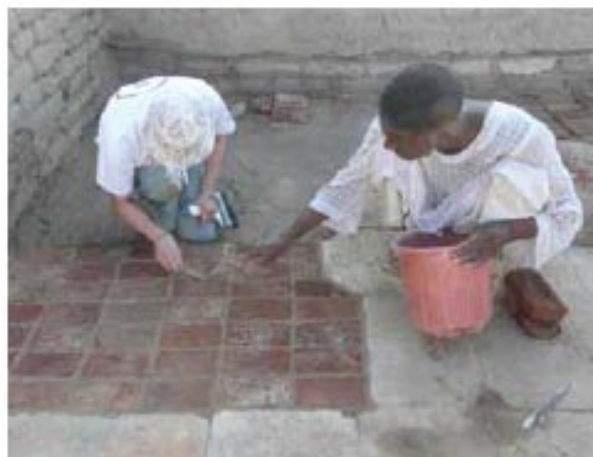
Fig. 6: Pointing the bricks.
