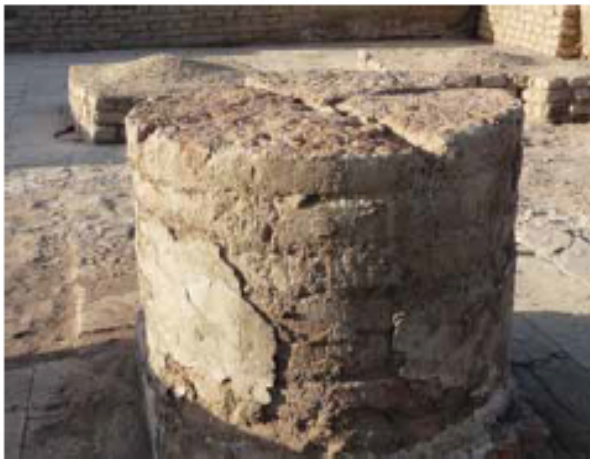
Fig. 13: Brick and lime rendered column, 2011.
