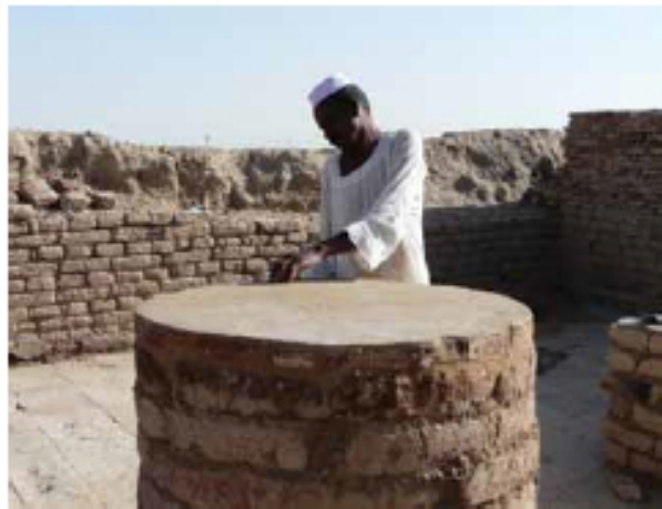
Fig. 14: Capping render to column, 2011.
