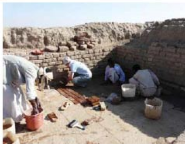
Fig. 5: Bedding the brick infill.
