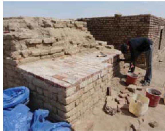
Fig. 9: Finished capped wall
