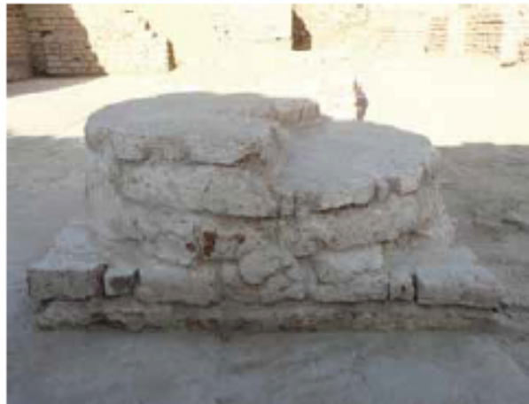
Fig. 12: Failed lime render to brick column.
