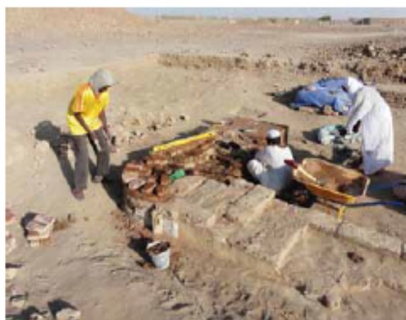
Fig. 15: Brick capping the Kiosk walls, 2011.
