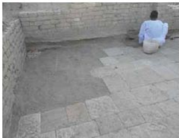
Fig. 4: Area of missing sandstone floor.
